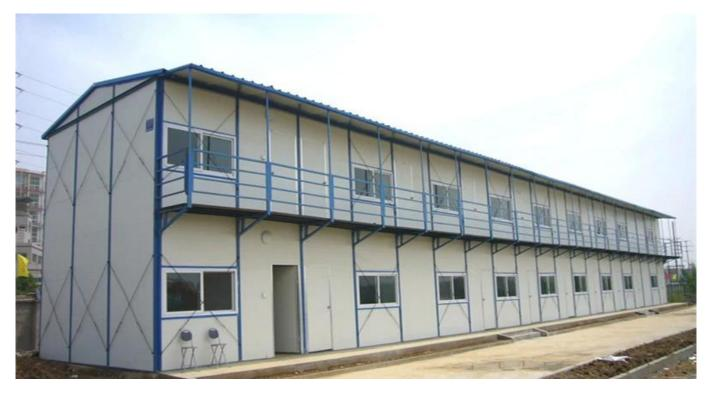
Place of Origin:Shandong, China (Mainland) Brand Name:QUALITY Material:Sandwich Panel Product name:Superior Quality <u>Prefab Dormitory</u> Modular Dorms Product:Steel Structure Prefab House Accessory:According to your request Roof&wall material:Sandwish Panel Structure:Steel Frame Size:Customized
